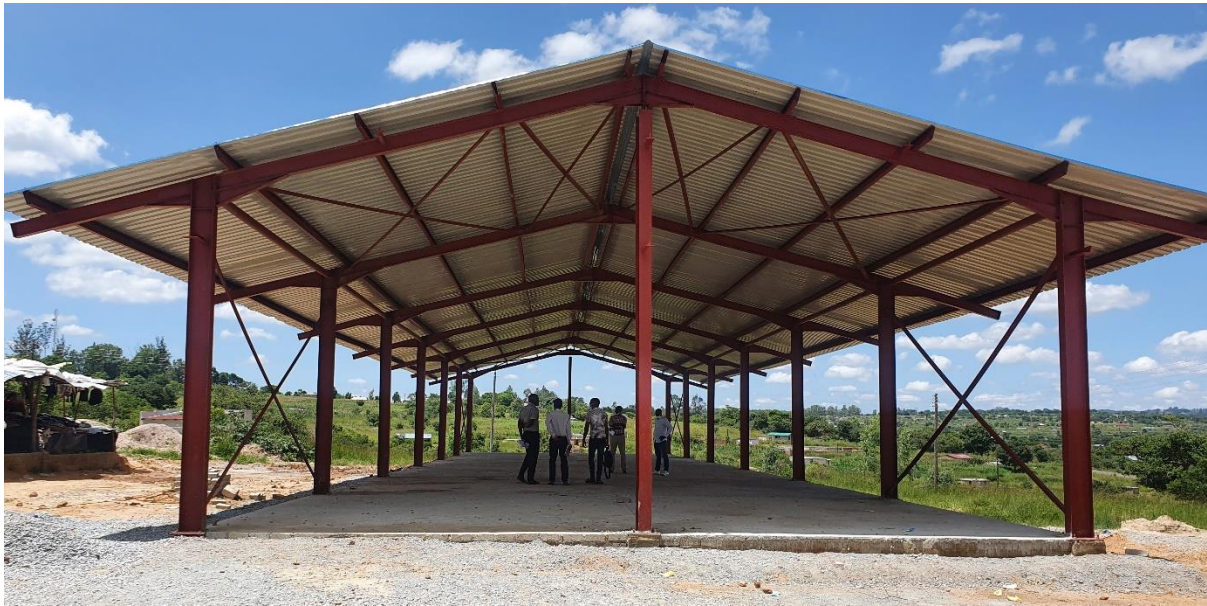
Figure 6: A shed constructed by the project in Goromonzi
